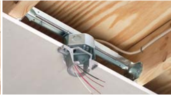
Attach to joists, adjust box position
