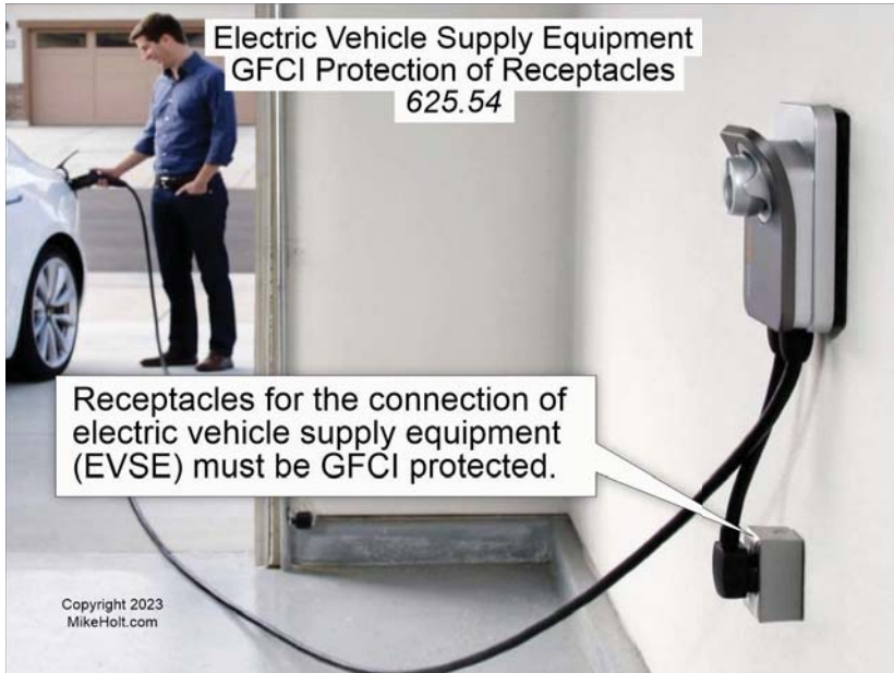
Fig. 3. All receptacles installed for the connection of EV supply equipment must be GFCI protected.
