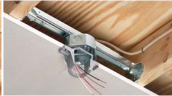
Attach to joists, adjust box position
