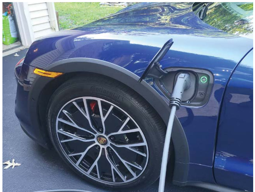
A Plus Electric installs Level 2 chargers for its residential clients in its service area.
