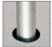
Insert conduit into sleeve.
