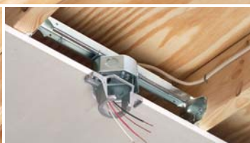
Attach to joists, adjust box position
