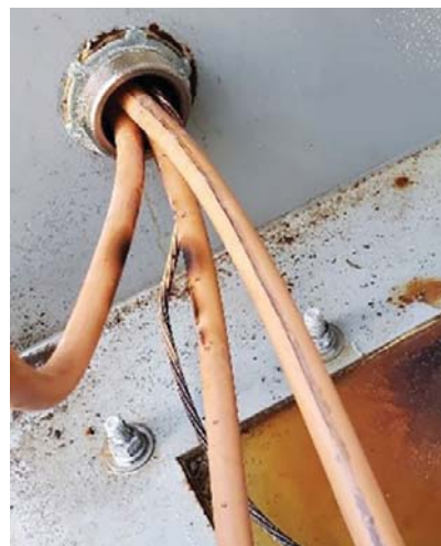
Photo 3. An example of damaged insulation.
