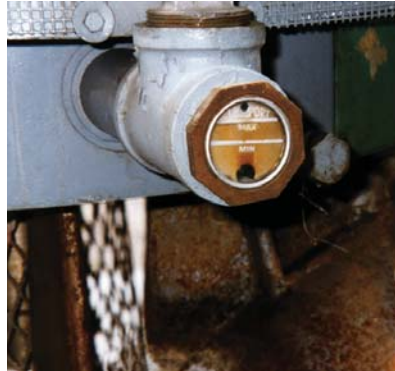
Photo 2. This is the oil sight glass for a vertical motor bearing.
