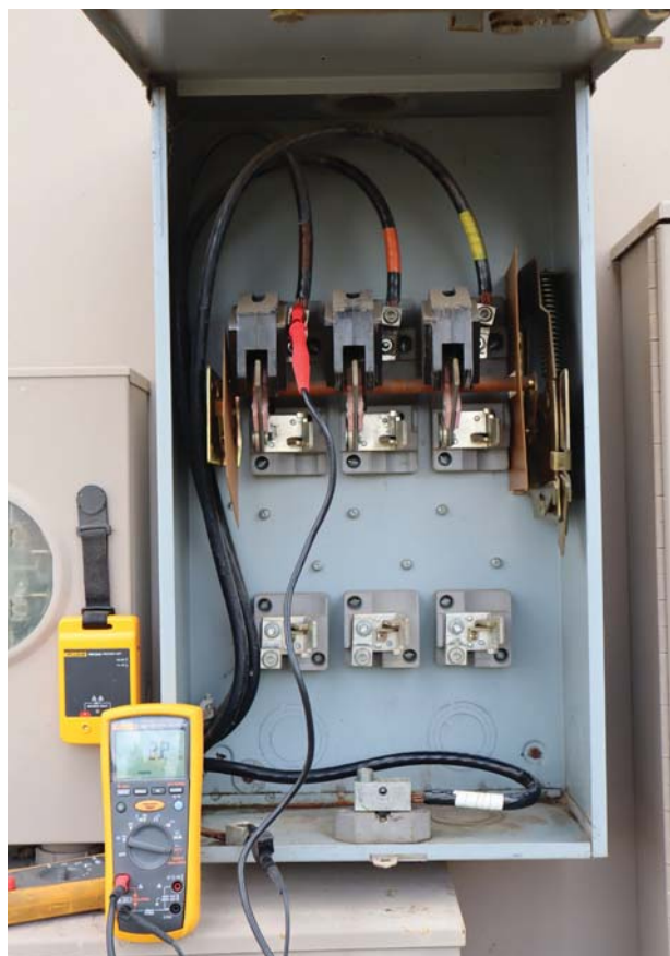
Fig. 4. The NEC Sec. 110.7 [Wiring Integrity] requires “completed wiring installations shall be free from short circuits, ground faults, or any connections to ground other than as required or permitted elsewhere in this Code.” Before installation of load side conductors into this 200A disconnect, the line side conductors are tested to ensure no ground faults exist. Load side conductors will be tested after installation.
