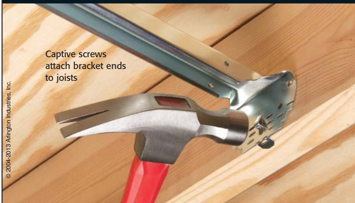
Attach to joists, adjust box position
