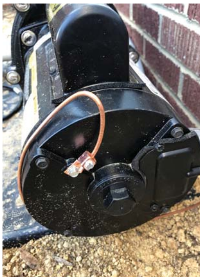
Bonding of metal parts of electrical equipment, per list item (6).
