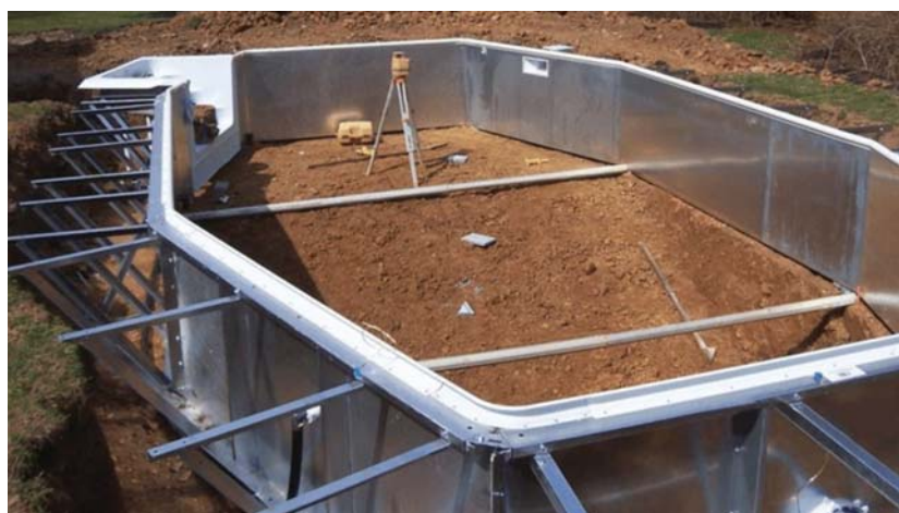
Structural metallic wall panel of a permanently installed pool, per list item (3).
