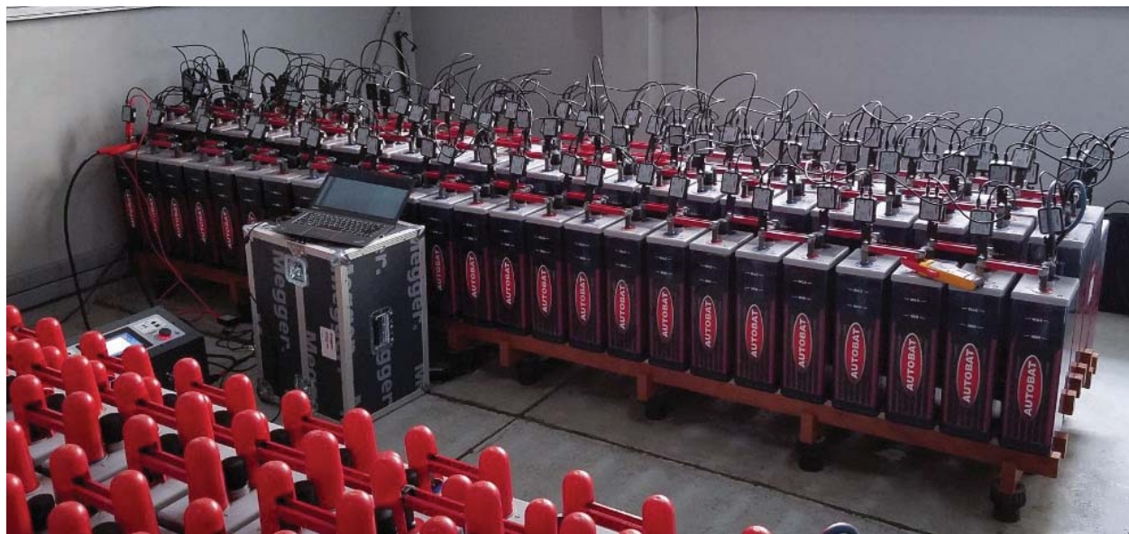
Photo 2. BVMs connected to all cells on the string provide individual cell-voltage values in real-time.
