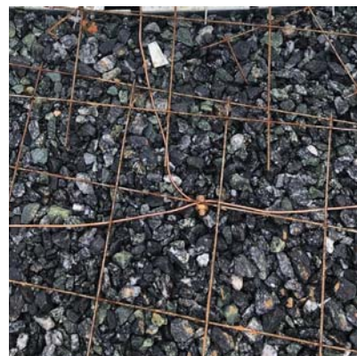
An 8 AWG copper conductor attached to perimeter surface structural reinforcing steel.
