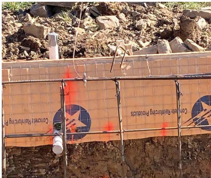
An 8 AWG copper conductor attached to the conductive pool shell. The other end of the conductor is to be attached to the perimeter surface structural reinforcing steel, copper ring, or copper grid.
