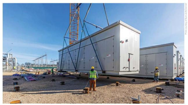
Workers set one of 122 battery containers at the Moss Landing battery energy storage site. Each container is home to 924 battery modules. The containers were engineered, pre-fabricated, and shipped from Pittsburgh, Kan. to Moss Landing, Calif., where they were set into place by Burns & McDonnell's self-perform construction team.
