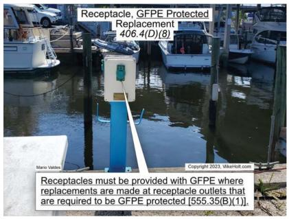
Fig. 2. Section 555.35(B)(1) contains requirements for GFPE protection of receptacles.
