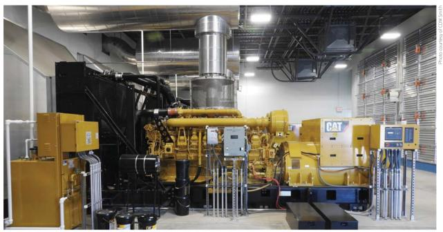
Emergency generators rated at 13.2kV that became operational in June 2022 at the Mark B. Whitaker Water Treatment Plant in Knoxville, Tenn. were the result of engineering and design work by Boston-based CDM Smith, a design partner in the facility's generator/electrical building upgrade project.
