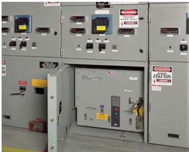
Photo 1. Designing out safety issues plays a large factor in reducing incidents. Notice the heavy-duty design of this cubicle door on arc-resistant switchgear. With all doors closed, latched, and bolted, an arc flash will be safely vented out the top of the switchgear with no danger to a worker standing in front of the equipment.
