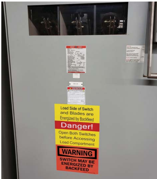
Labels that clearly warn workers of hazards inside equipment are an example of the Awareness Risk Control Method.
