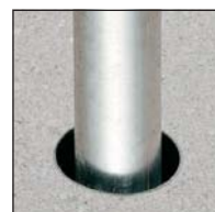
Insert conduit into sleeve.
