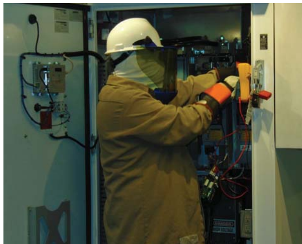
Photo 3. Verifying an electrically safe work condition is considered working on live parts because components may still be energized. Most workers experience some uneasiness working on energized circuits as they should. PPE is generally not comfortable to wear. What else could the worker be thinking about during this task?
