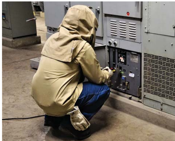
Photo 2. Installing a remote racking motor on a 480V low-voltage power circuit breaker is a common task that exposes workers to potentially a severe arc flash hazard. The domino effect could come into play: The work area is hot and uncomfortable; the hood makes it hard to breathe, and fog may accumulate on the face shield, making it hard to see. The breaker location on the bottom row is not an easy place to work. Frustration getting the motor to latch on the breaker could abruptly move the breaker enough to allow unmaintained equipment to fail and produce an arc flash. The worker does not have his arc-rated shirt tucked in which should have been addressed in the job briefing. What other pressures, concerns, or physical impairments may be affecting this worker?
