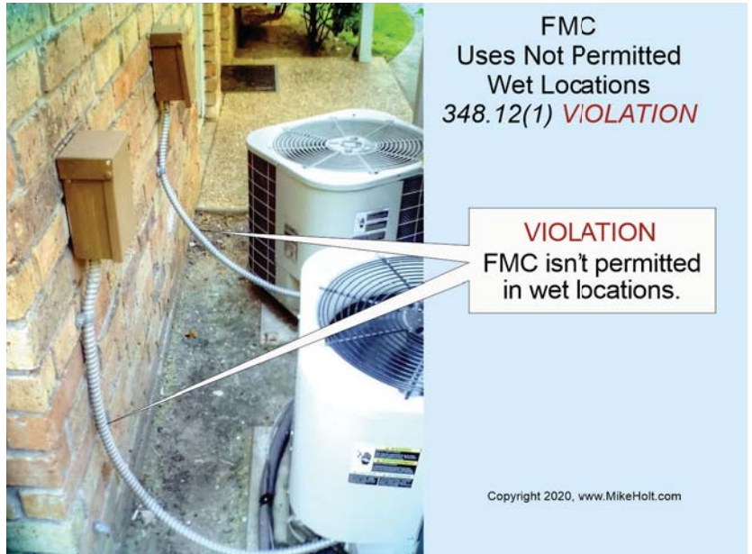
Fig. 2. FMC is primarily used where equipment moves or vibrates, although it's not permitted in wet locations.
