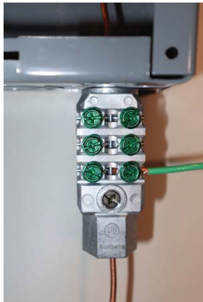
Photo 3b. NEC Sec. 250.94 requires bonding for communication systems. One of the two options is the use of an Intersystem Bonding Termination (IBT) device. This IBT bonds communication wiring (green conductor) to the grounding electrode conductor at the service exterior to the service enclosure.
