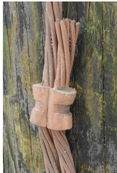
Photo 3c. An irreversible crimp connector has been applied by compression to these stranded grounding conductors.
