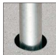
Insert conduit into sleeve.
