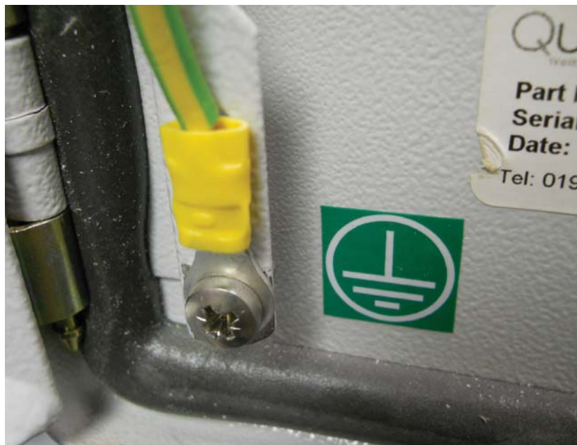
Photo 4. Here’s an example of “connections that are part of a listed assembly.” Panel makers will often identify termination points for the location of grounding and bonding connections. Notice the listed tool-cripped connector with the yellow plastic covering to identify AWG size for the connector. Additionally, the grounding symbol indicates the proper location for this bonding connection.
