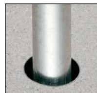
Insert conduit into sleeve.
