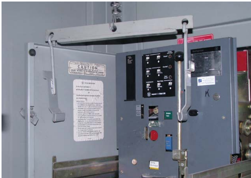
Photos 3a and 3b. This circuit breaker is ready to be lifted from its extension arms.
