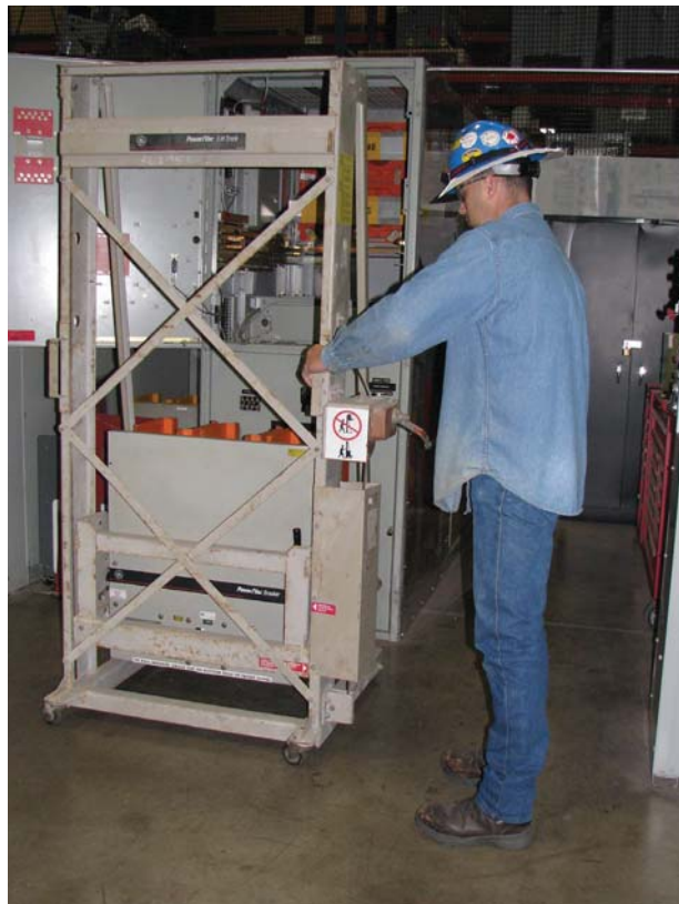
Photo 4b. This technician is using the lifting platform to install a medium-voltage draw-out type vacuum circuit breaker.
