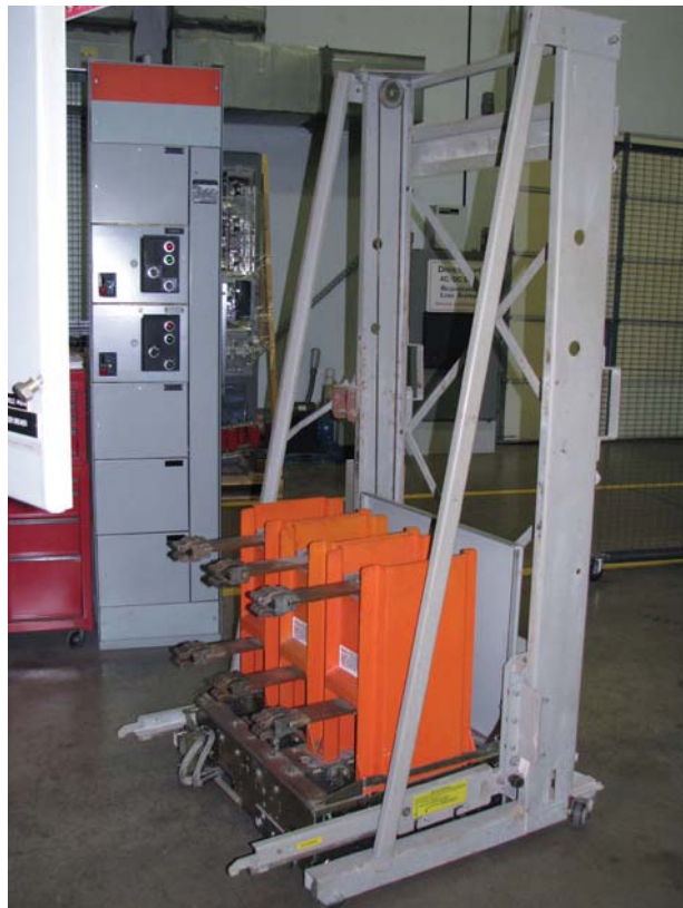
Photo 4a. Here's an example of a vacuum circuit breaker lifting platform.
