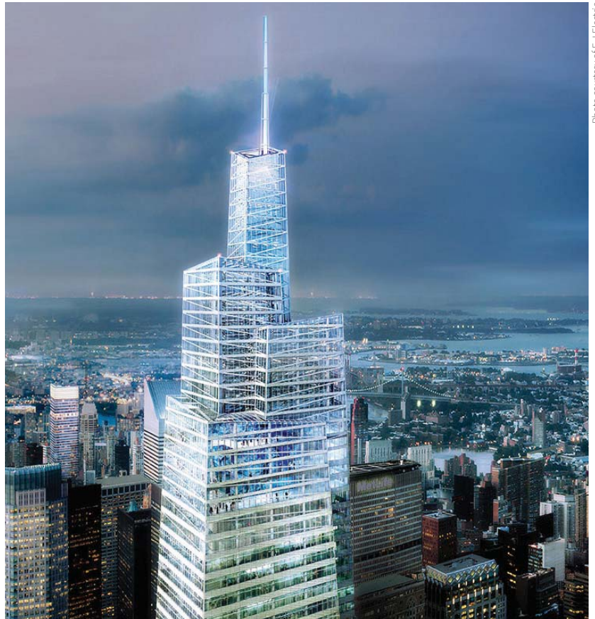
Photo courtesy of E-J Electric
