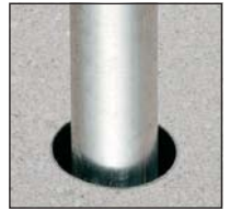
Insert conduit into sleeve.
