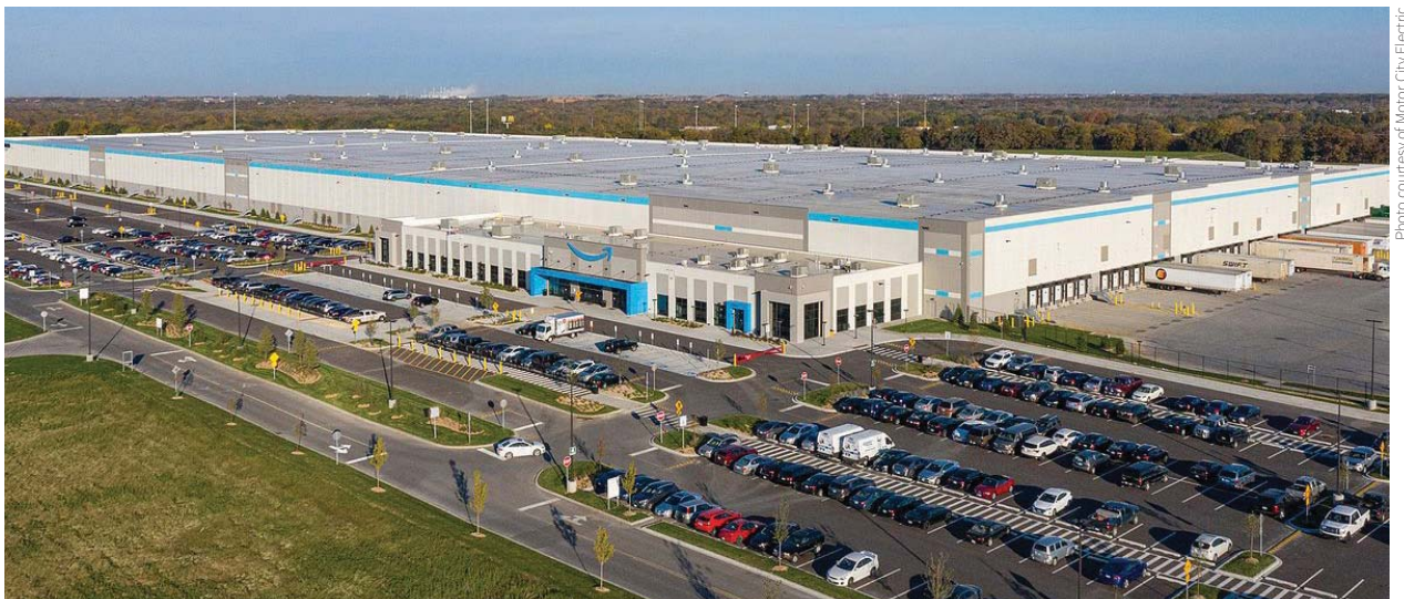
Photo courtesy of Motor City Electric
