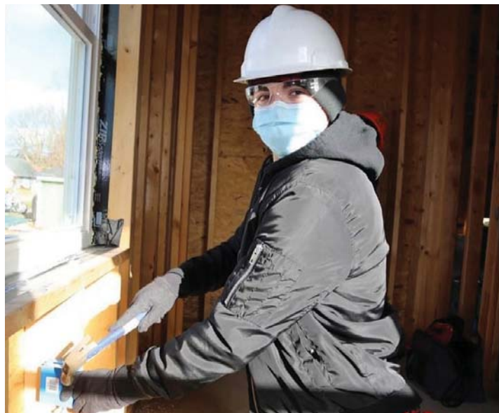
Dale Wolgamuth, who graduated in June 2022, is hammering in new work PVC boxes for receptacle and switch locations.
