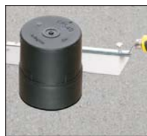
After concrete sets, cut sleeve flush with surface.
