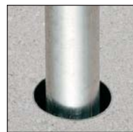
Insert conduit into sleeve.
