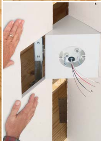
Position box between framing members by sliding it along the expandable brackets
