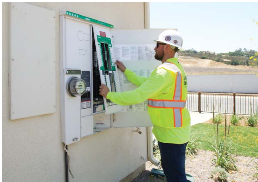
An electrician installing an energy center system
