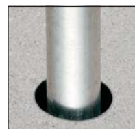
Insert conduit into sleeve.
