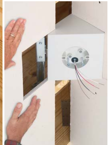
Position box between framing members by sliding it along the expandable brackets
