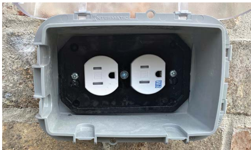
Photo 1. A close-up view of a receptacle that employs a weather-resistant (WR) rating.
