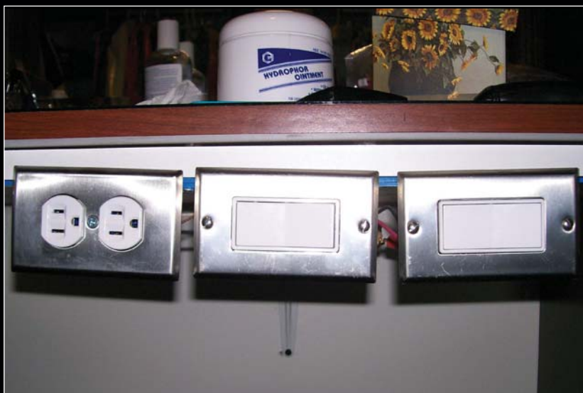
Photo 1. If you look closely between the boxes, you can see the exposed conductors.
