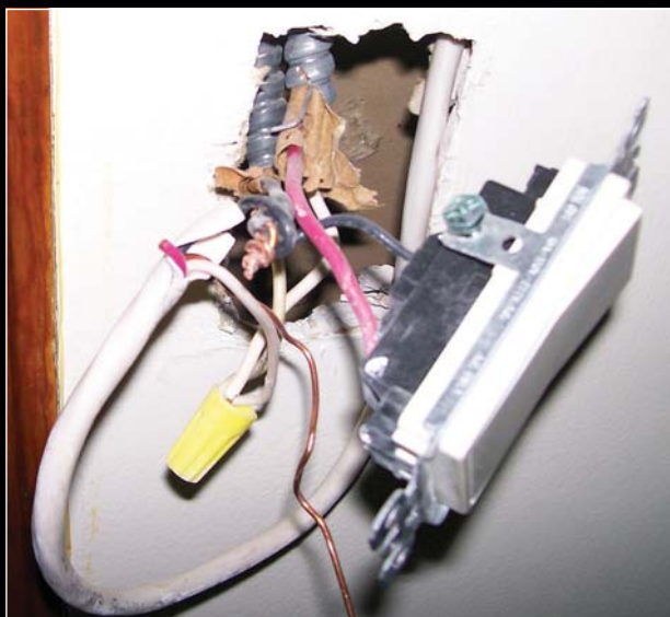
Photo 8. There is so much more room for splices when you don't use a box!
