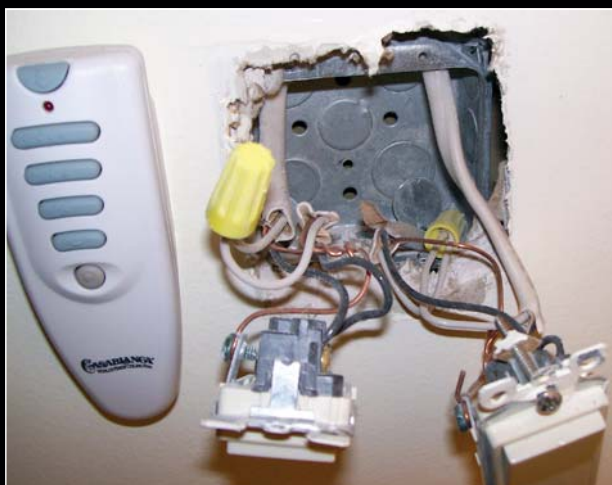
Photo 9. At least the installer used a box here! Nice job with the grounding as well.
