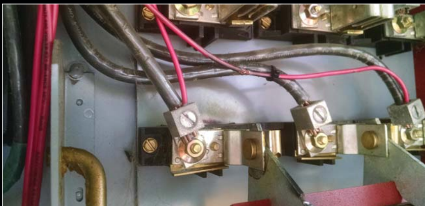
Photo 17. Notice the damaged blade on the switch and the burned wire where it crossed phases.
