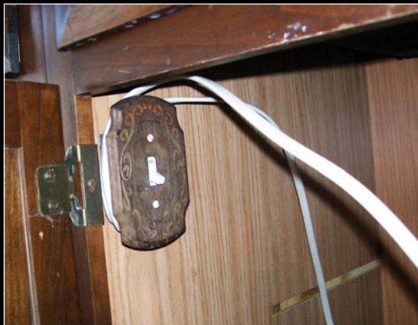
Photo 10. Notice the NM cables wrapped around the box and stretched across the cabinet.
