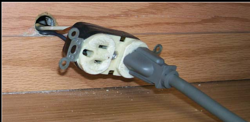
Photo 12. Apparently, the installer didn't have a box to cut in.
