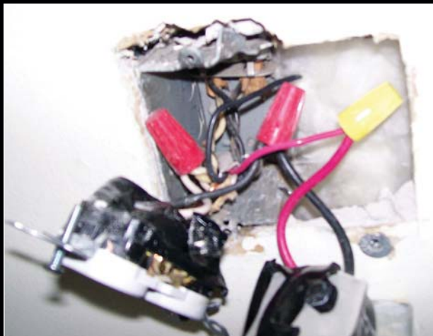
Photo 7. Removing the devices revealed the hacked apart 1-gang box and the installer's method of wiring the thermostat.
