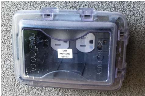
Photo 2. A weather-resistant (WR) receptacle located in a wet location based on the protection afforded by the in-use extra-duty cover.
