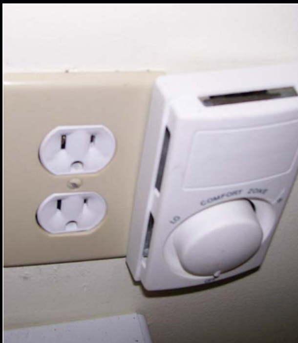
Photo 6. This thermostat didn't sit flush against the wall, indicating some issue.
