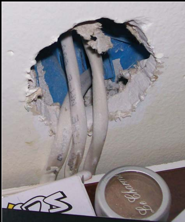
Photo 3. A view of the NM cables that are pinched behind the countertop.
