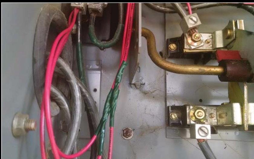
Photo 16. A closer look reveals grounding issues as well as water entering the enclosure.
