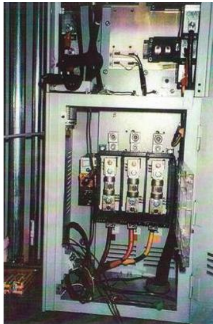
Photo 1. The open electric cabinet with three phase conductors feeding in from the floor. Plastic acrylic block is opened to expose three fuses limited to 125A per phase. Left of fuses is the clock wire that bypasses the safety interlock. In the top of the picture is the beginning electronics of the VFD.
