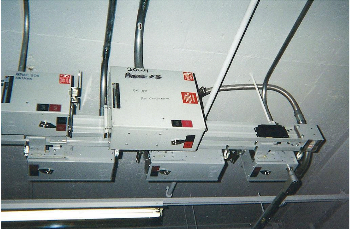
Photo 3. This overhead safety switch is connected to the VFD. It is located too far away to be of any advantage in this accident.
