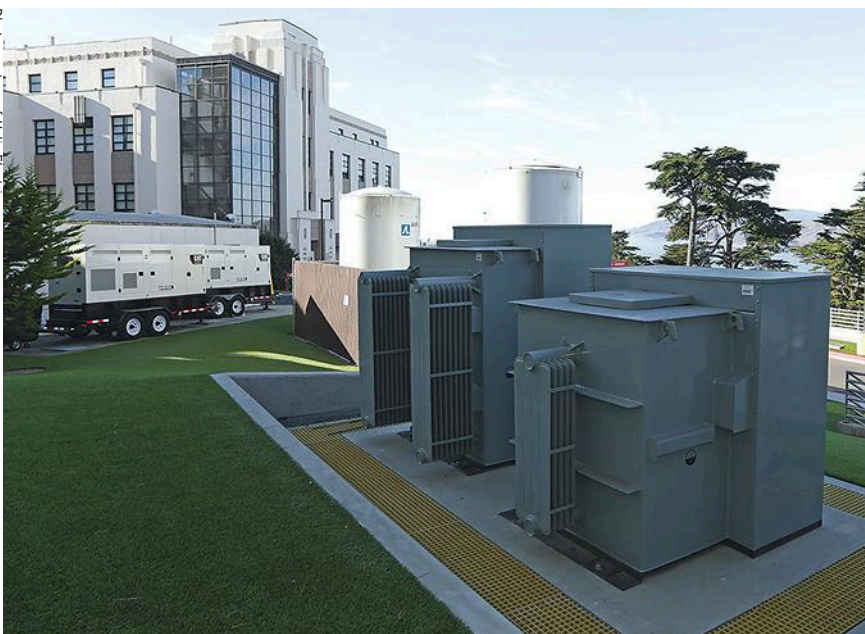
Helix Electric installed two new transformers as part of the 12kV A/B underground distribution system upgrade at the San Francisco Veterans Administration Medical Center.
