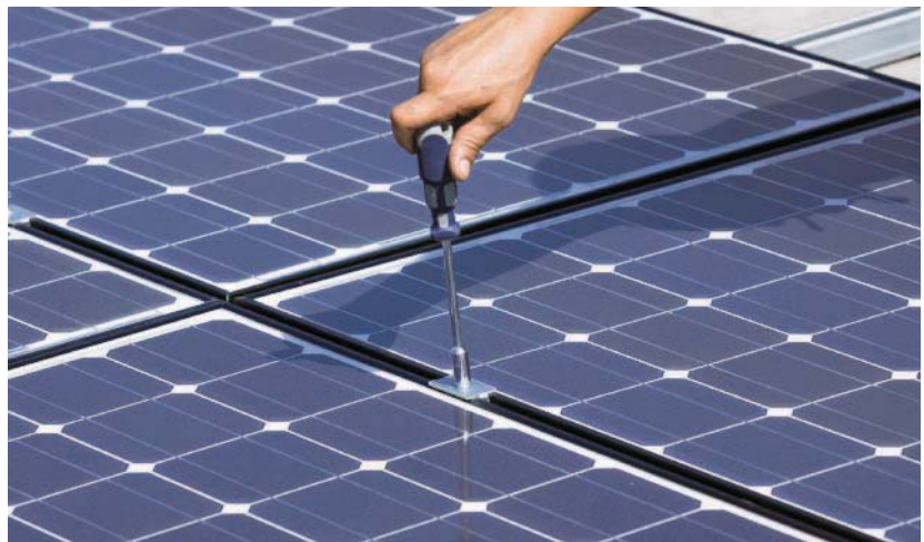
The installation of racking components has been a heated point of discussion.
